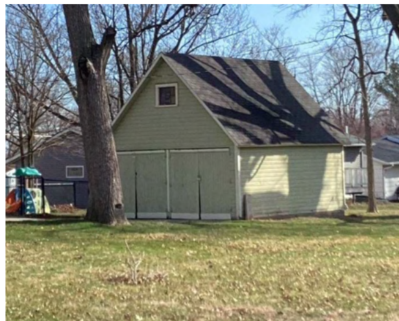
Figure 74: Example of outbuilding with features that should be preserved.
