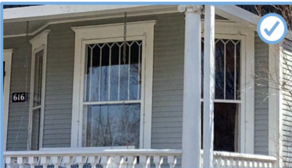
Figure 62: Example of storm windows appropriately installed to preserve historic windows.
