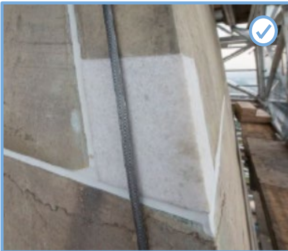
Figure 29: Appropriate Dutchman Repair on Masonry.
