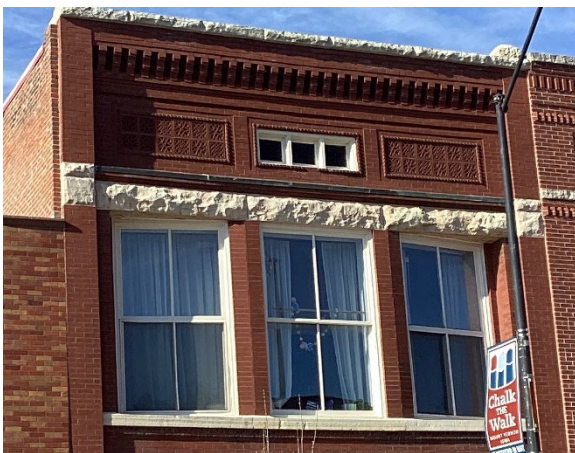
Figure 112: Example of upper story windows on a historic storefront.
