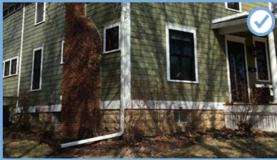
Figure 50: Example of appropriate gutter with downspout leading away from the building.
