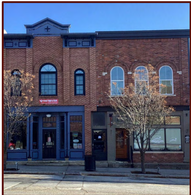
Figure 3: The revitalization of historic downtown buildings can act as a major draw for entertainment and activity.
