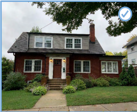
Figure 78: Appropriate side addition that is compatible in its massing, scale, and proportions.
