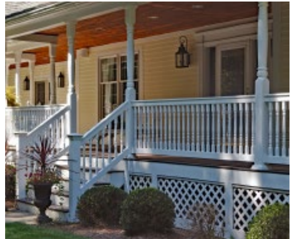
Pressure treated lumber balustrade and railing.
