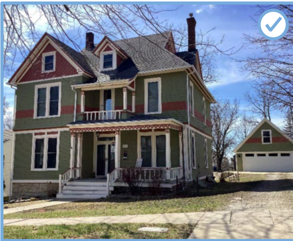
Figure 80: Example of appropriate new accessory structure, located at the rear of the property and is consistent with the historic residence.
