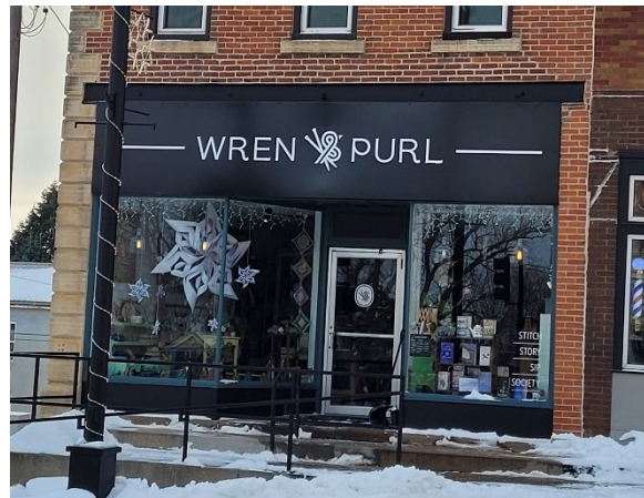
Figure 102: Example of typical two-part commercial block building in Mount Vernon's Commercial District.
