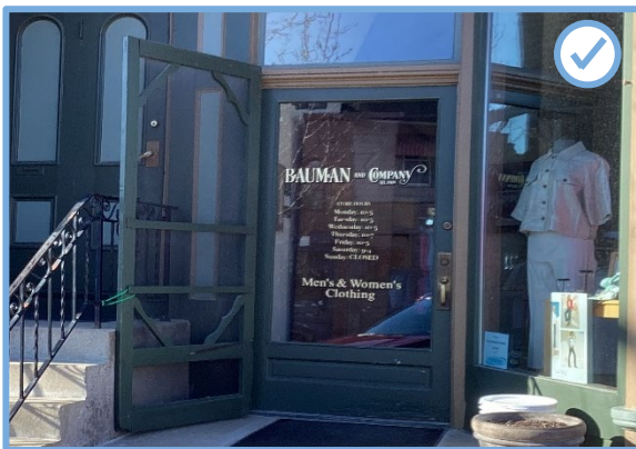
Figure 106: Example of screen door on storefront entrance.
