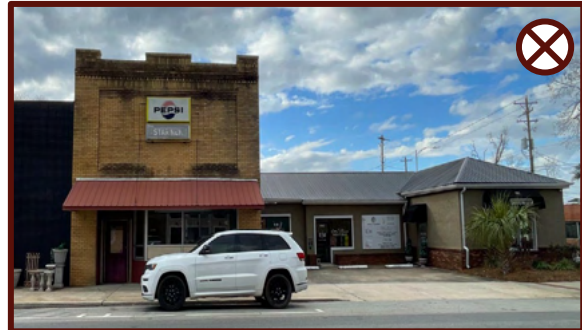
Figure 119: Inappropriate new commercial construction with incompatible setback, massing, and fenestration.
