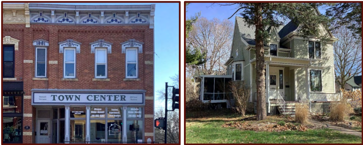
Figure 22: These examples of properties with moderate historic integrity have all retained their form, but some materials and some stylistic details have been lost or changed, in this case the windows and enclosed porch addition.
