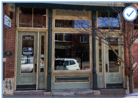
Figure 105: Example of typical commercial doors and storefront in Mount Vernon's Commercial District.
