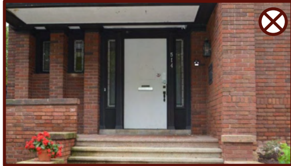
Figure 58: Example of inappropriate front door replacement.
