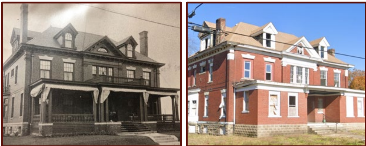
Figure 20: Before (left) and after (right) example of how the loss of building's character-defining details, in this case the removal of a residence's original cornice dentils, windows, part of the chimney stack, and enclosing its porch, damages the character of a historic building.
