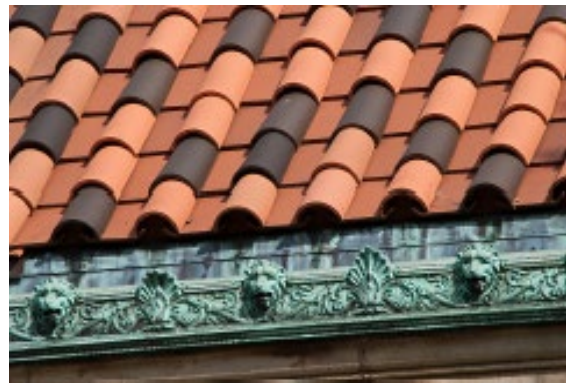
Clay tile roofing.
