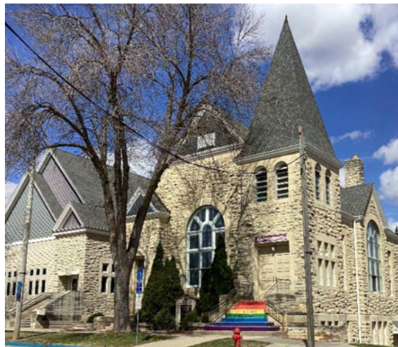
Figure 92: Complex rooflines should be preserved and taken into consideration when repairing or replacing elements
