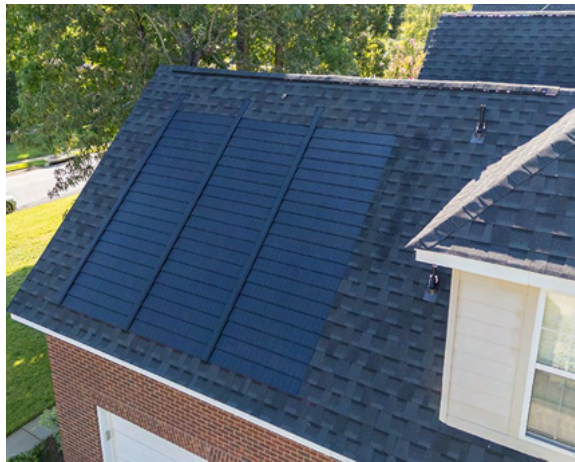
Figure 72: Example of integrated solar shingles.
