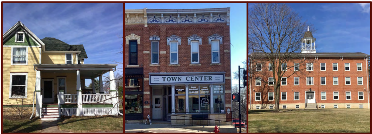
Figure 10: From left to right: Typical residential, commercial, and institutional building types found in Mount Vernon's historic districts.
