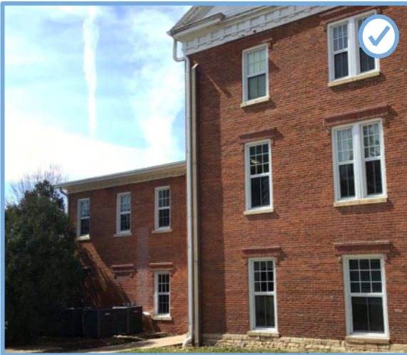
Figure 96: Appropriate gutter located on an inconspicuous location.
