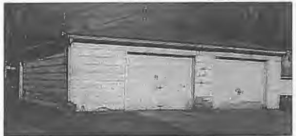
Inappropriate siding and roof pitch
