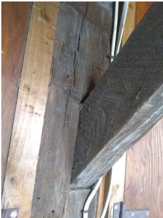
Figure 13. Details of barn/garage interior showing hewn posts and beams and sawn bracing. Photographs taken by Caroline Kelly, March 2019.
