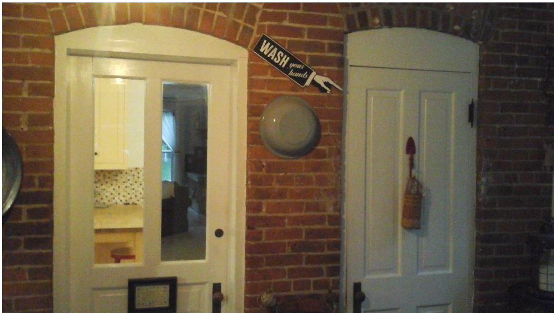
Figure 8. Interior views of the Pease House. Top: example of interior moldings including segmental arch over interior doorway. Bottom doors into the kitchen addition on the rear of the house. These doors are underneath the later frame enclosed porch addition. Photographs taken September 2018.
