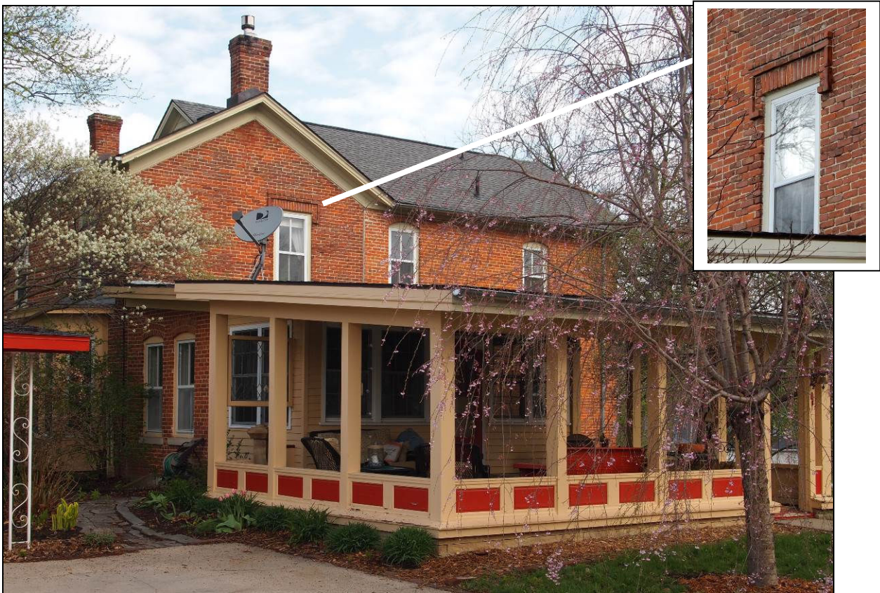
Figure 3. Rear of the Pease House showing the U-shaped brick-corbelled lintel on the second story window (inset detail). View is looking NNW. Photograph taken May 4, 2018.
