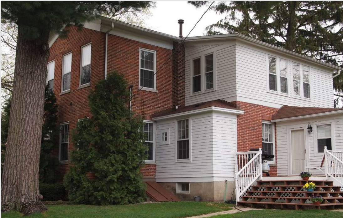
Figure 6. Rear and north side of Knott House looking South. Photograph taken May 4, 2018.
