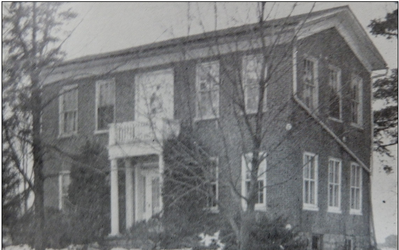
Figure 14. Photograph of the Knott House published in the Mount Vernon Centennial book in 1948. The actual date of this photograph is not known. Note that the 2/2 “windows” visible on the gable end are storm windows covering the original 6/6 windows. Source: Centennial Committee 1948
