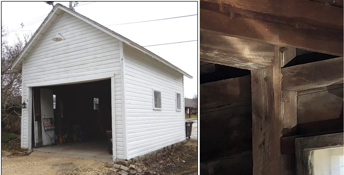
Figure 11. Left: Detached barn/garage looking West; Right Detail of interior framing showing mortise-and-tenon pegged joinery. Photograph taken March 30, 2019.
