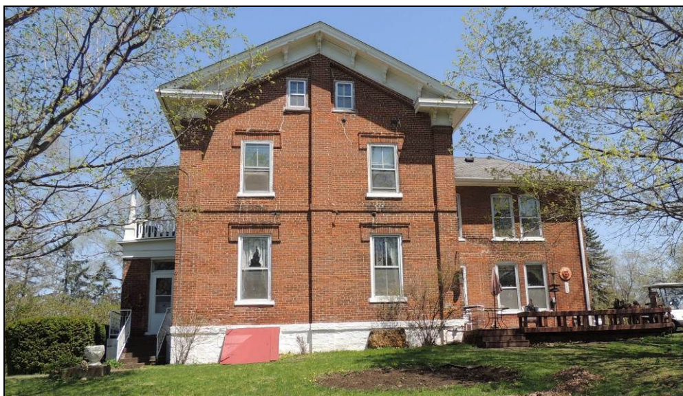
Figure 3. South side. Photograph taken May 4, 2018.
