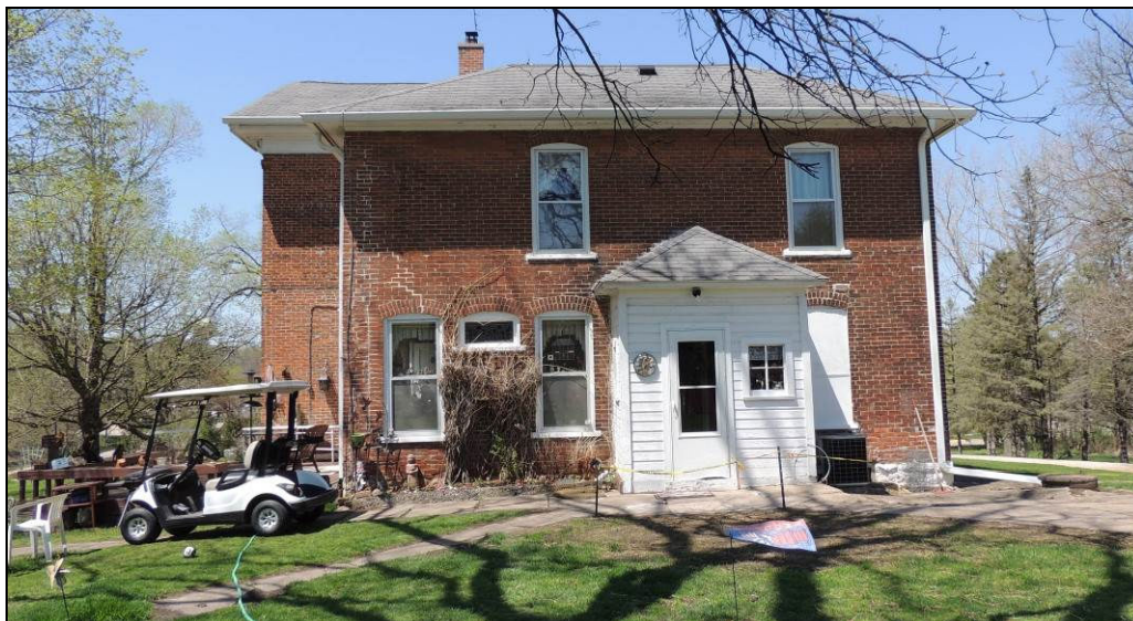
Figure 5. Rear (east side) of house. Photograph taken May 4, 2018.
