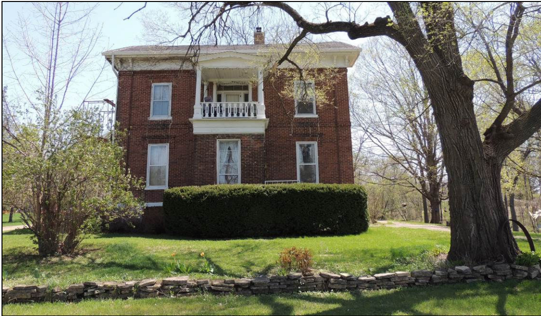
Figure 2. Façade (west side). Photograph taken May 4, 2018.
