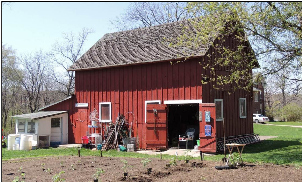
Figure 10. Barn, east and north sides. Photograph taken May 4, 2018.
