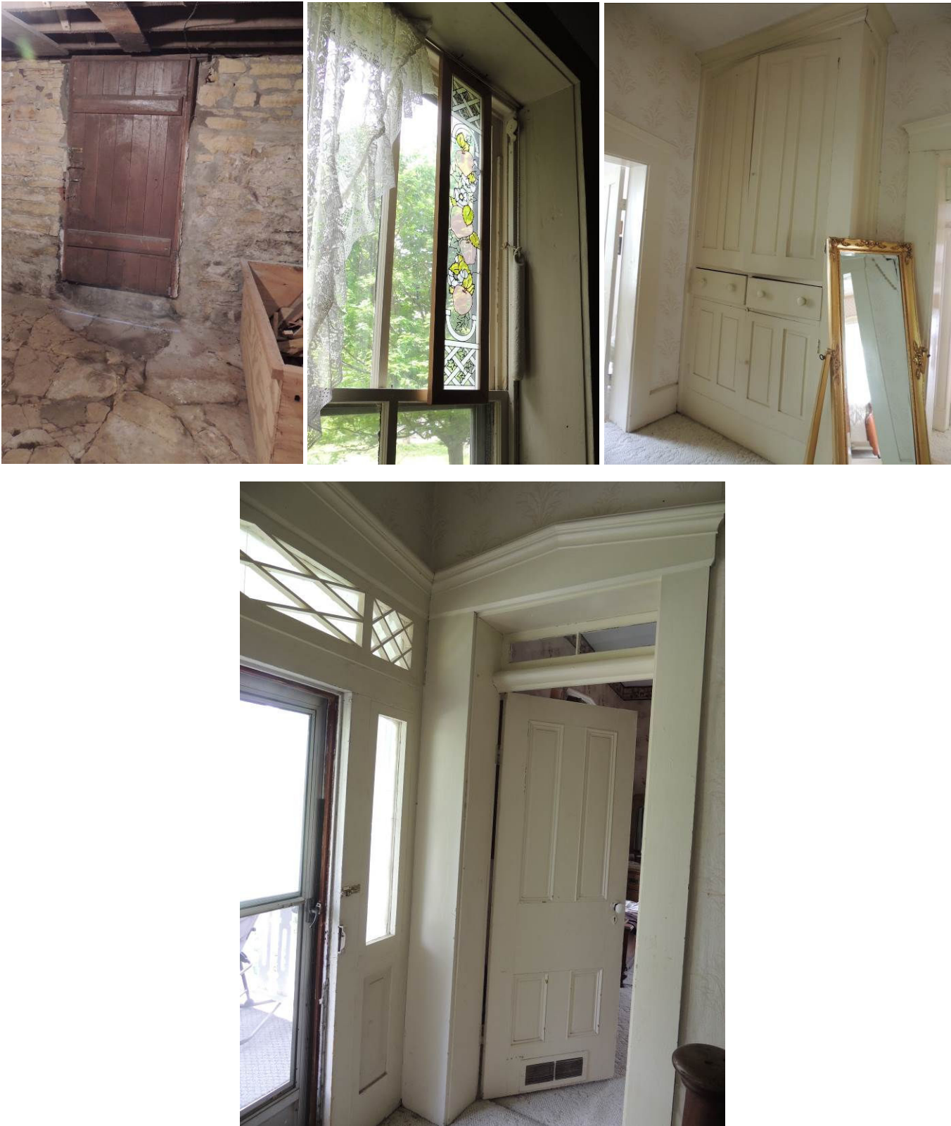
Figure 8. Interior views (clockwise from top left): flagstone floor in cellar; sash weight on outside of window casing on the interior; built-in cabinet/drawers in the upstairs hallway; and balcony door (to left) and door with peaked lintel just inside balcony door (to right). Photographs taken May 2018.
