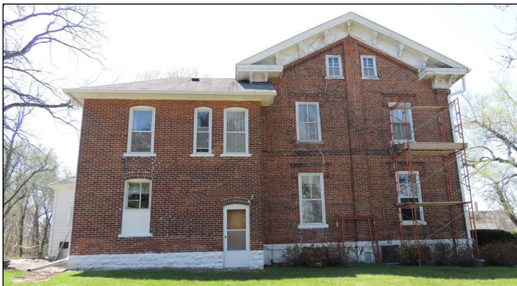
Figure 6. North side. Photograph taken May 4, 2018.
