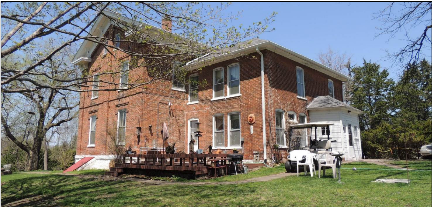
Figure 4. Southeast corner of house. Photograph taken May 4, 2018.
