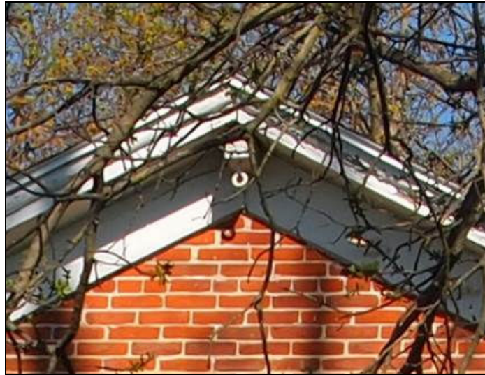
Figure 6. Hardware for block and tackle at gable peak on rear (east side) of Smith House. Photograph taken May 4, 2018.
