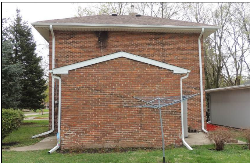
Figure 9. West (rear) side of 303 A Avenue SE looking ESE. Photograph taken May 2, 2018.
