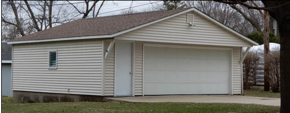
Figure 14. Modern garage behind 303 A Avenue SE looking South. Photograph taken March 30, 2019.
