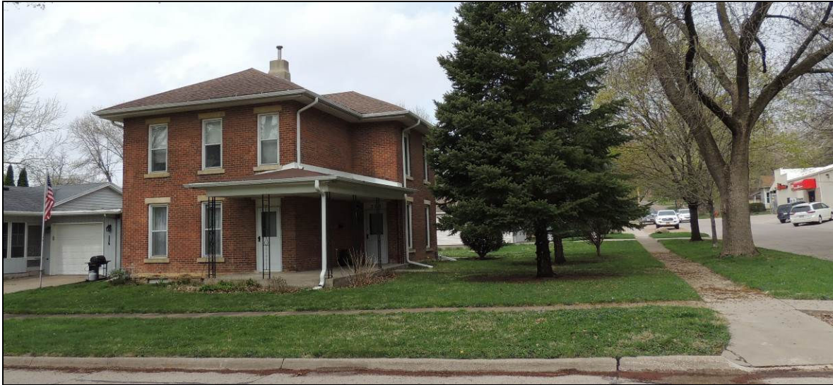
Figure 1. 303 A Avenue SE looking west. Photograph taken May 2, 2018.
