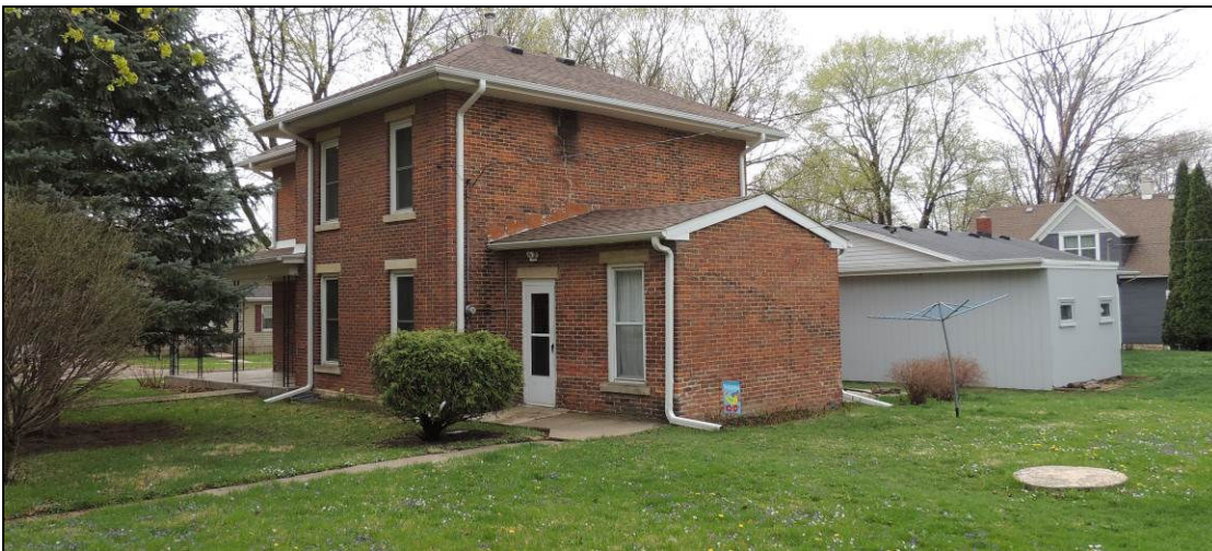
Figure 8. North and west sides of 303 A Avenue SE looking South. Photograph taken May 2, 2018.
