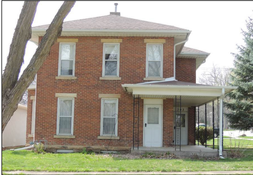
Figure 6. Façade of 303 A Avenue SE looking NW. Photograph taken May 2, 2018.
