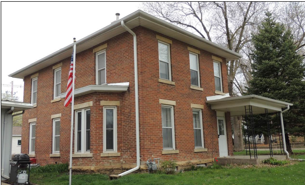
Figure 11. South and east sides of 303 A Avenue SE looking North. Photograph taken May 2, 2018.
