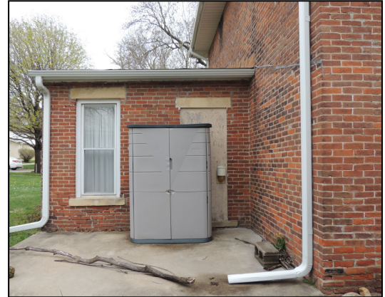
Figure 10. South side of rear structure looking NE. Photograph taken May 2, 2018.
