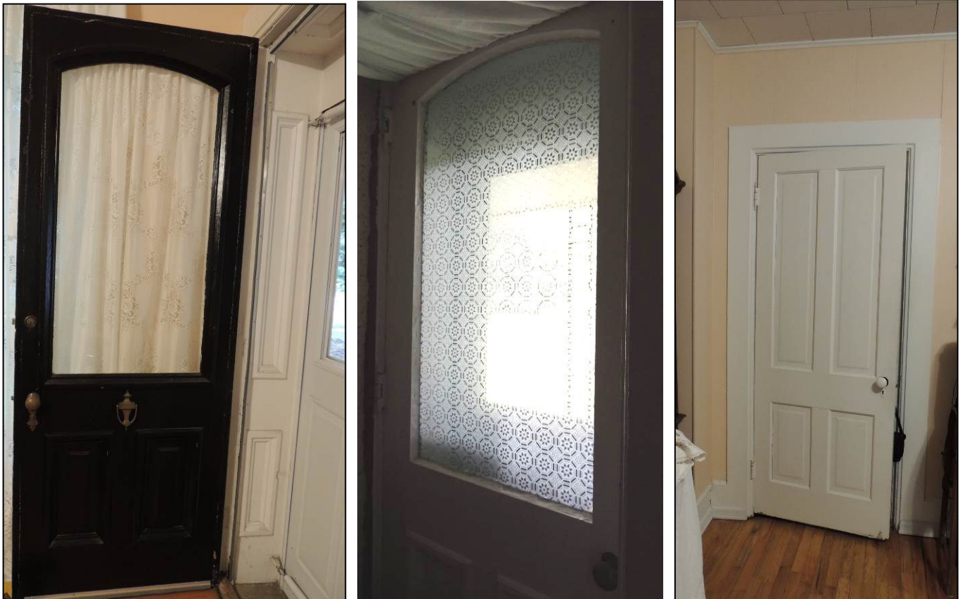
Figure 13. Interior views of the front door off the NE porch (left), the original front door on the east side of the house (center), and an interior 4-paneled door also showing original woodwork and a porcelain doorknob. Photographs taken June 22, 2018.
