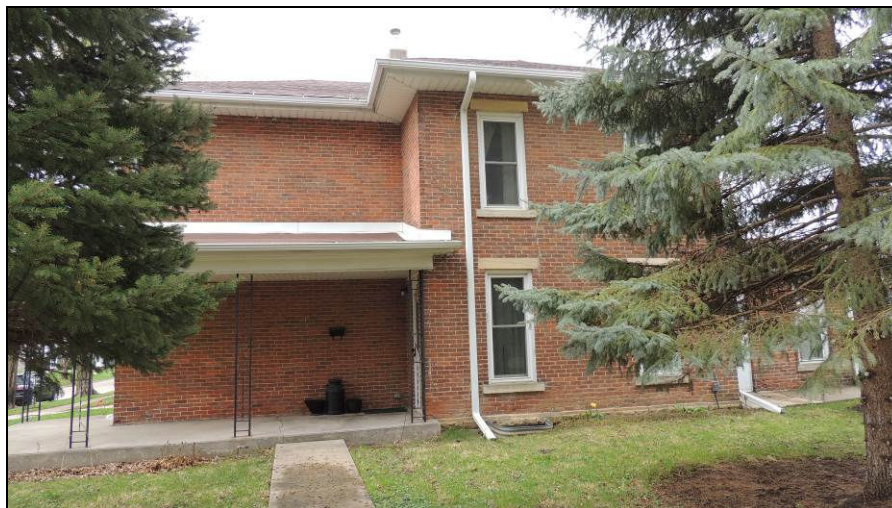
Figure 7. North side of 303 A Avenue SE looking SW. Photograph taken May 2, 2018.
