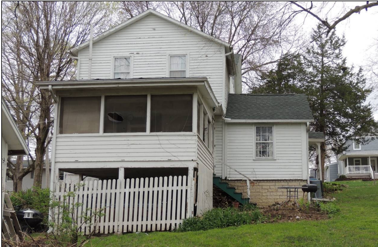
Figure 4. Rear of McCartney House looking NNE. Photograph taken May 2, 2018.
