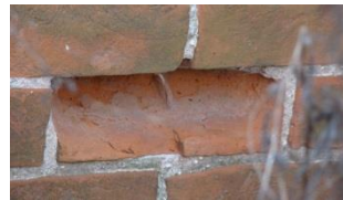
Brick damaged from pecking
